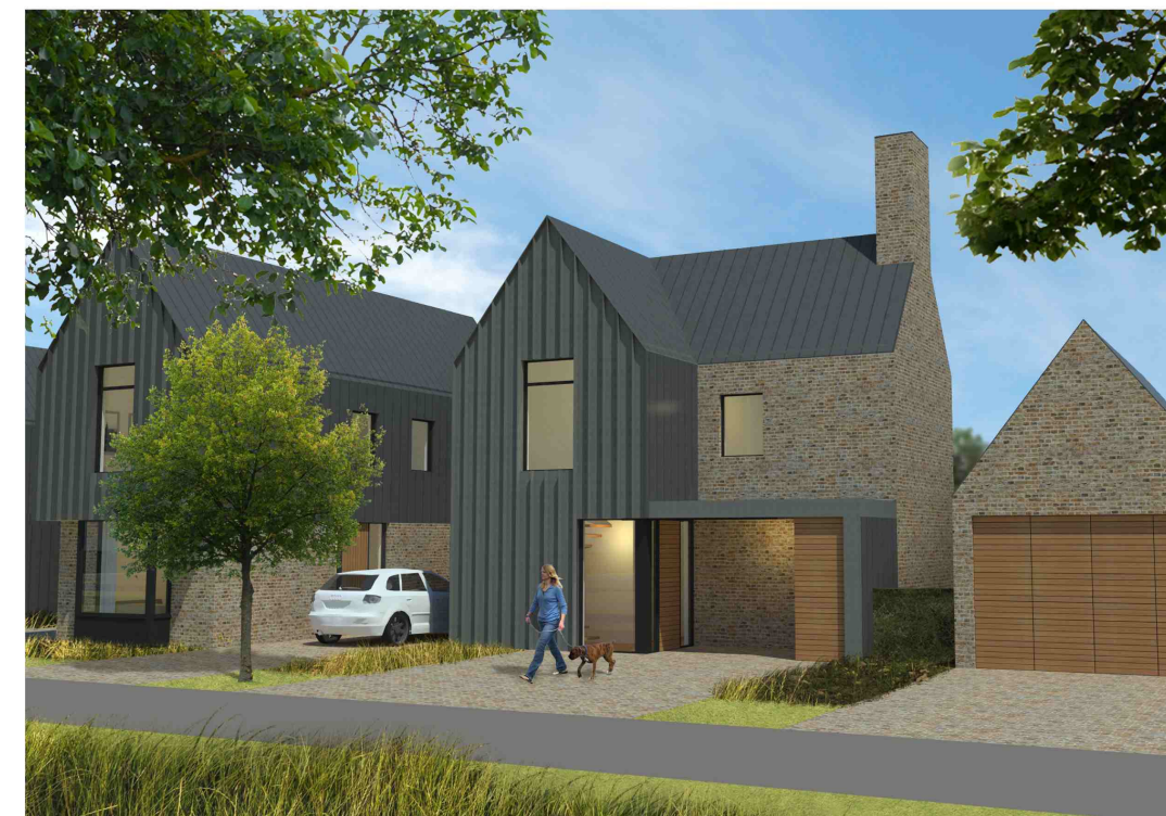
TW-A.1 Street Elevation Location specific materials. Zinc roof and vertical cladding, brickwork and timber details
